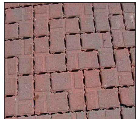
Figure 2.11.7 Pervious Interlocking Concrete Pavement
