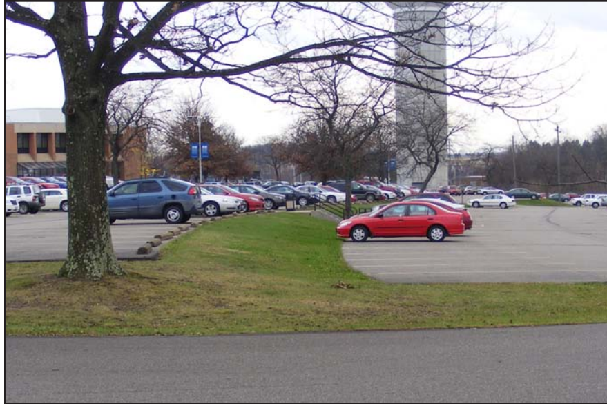
Figure 2.11.3 Terrace sloping areas to limit the pavement slope (photo credit: Brandon Andreson).
