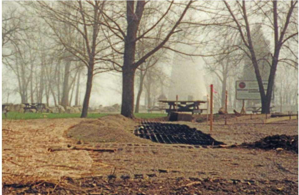
Pervious Paver installation
