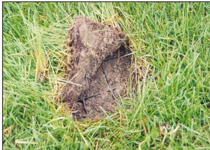
Figure 2.11.9 Vegetated Grid System with established turf grass.
