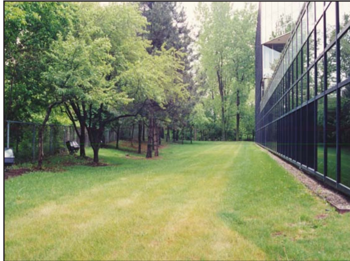
Figure 2.11.8 Vegetated Grid System utilized for fire access.
